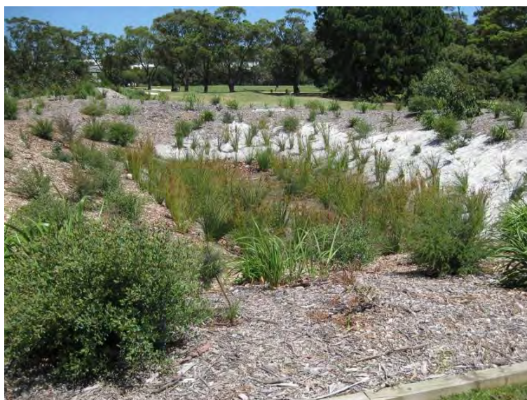
Plate 6-2 Example of a bio-retention basin at Manly Golf Course
