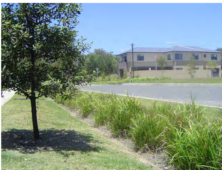
Plate 6-1 Example of a bio-retention swale at Warriewood
