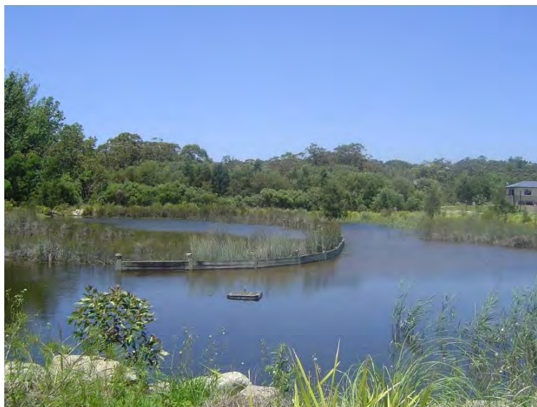
Plate 6-3 Example of a constructed wetland at Warriewood
